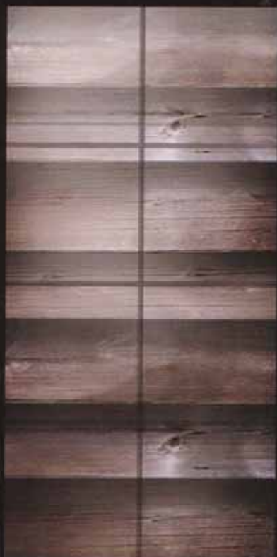
Stairs [wooden and stone]
